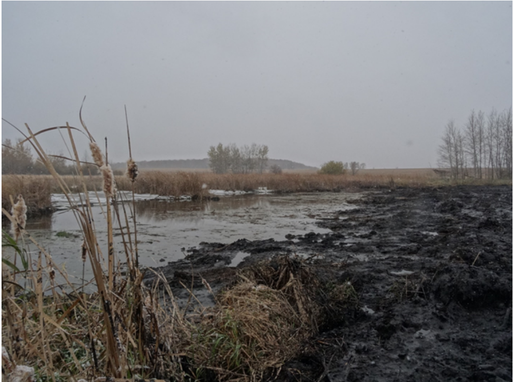
The completed scraping of the non native vegetation for the wetland restoration area.
