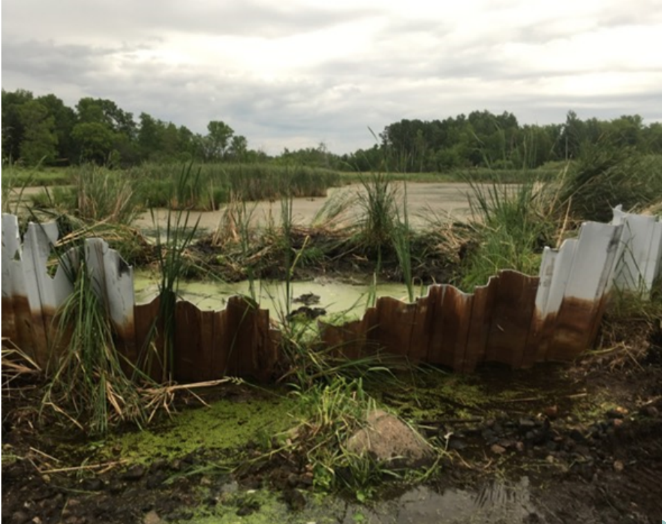
The original weir structure.
