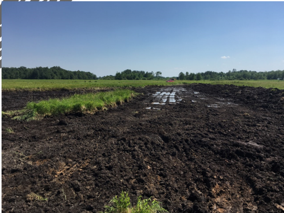
The completed scraping of the non native vegetation for one of the wetland restoration areas.
