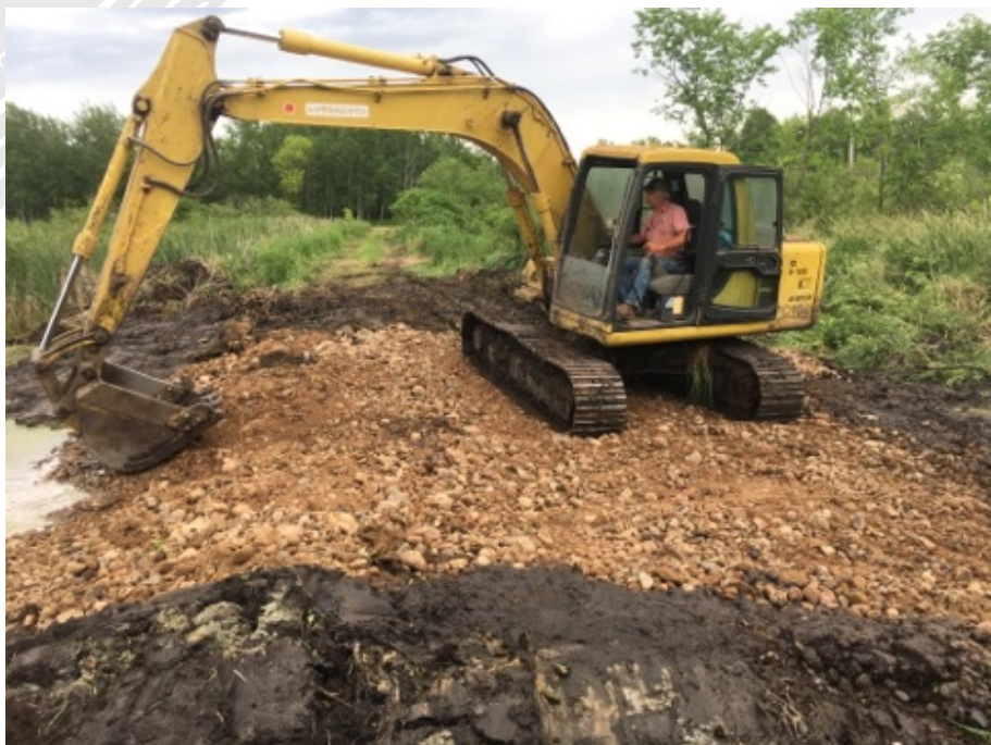
The new weir structure that was installed with the rock spillway installed over the top.
